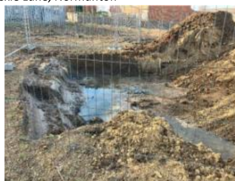
Figure B - Shallow spent oxide contamination excavation at Buckle Lane, Normanton.
