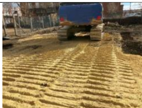
Figure C - Excavation areas having been backfilled with imported suitable for use material.
