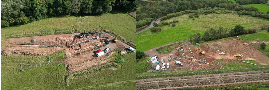
Figure 9 River Caldew diversion construction sites
