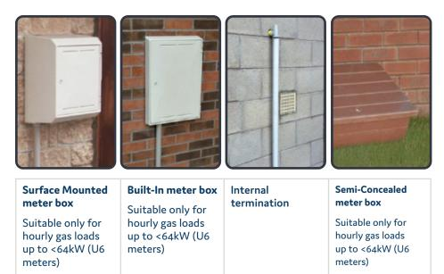
Northern Gas Networks will supply surface mounted or semi concealed meter boxes. If you require a built-in box, you or your builder will need to supply this and build it into your wall. Northern Gas Networks do not fit gas meters - you will need to contact your preferred gas supplier and arrange for them to fit a meter to your new gas supply.
