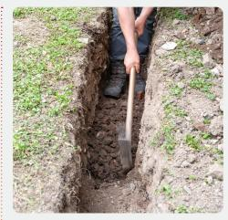
you will need to dig down another **75mm** and fill this with fine material so we can lay the pipe on top of it.
