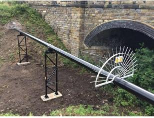
To re-life the asset the pipework and support structure is blasted and re-coated to current specification, new pipe cradles installed, and additional security put in place.
