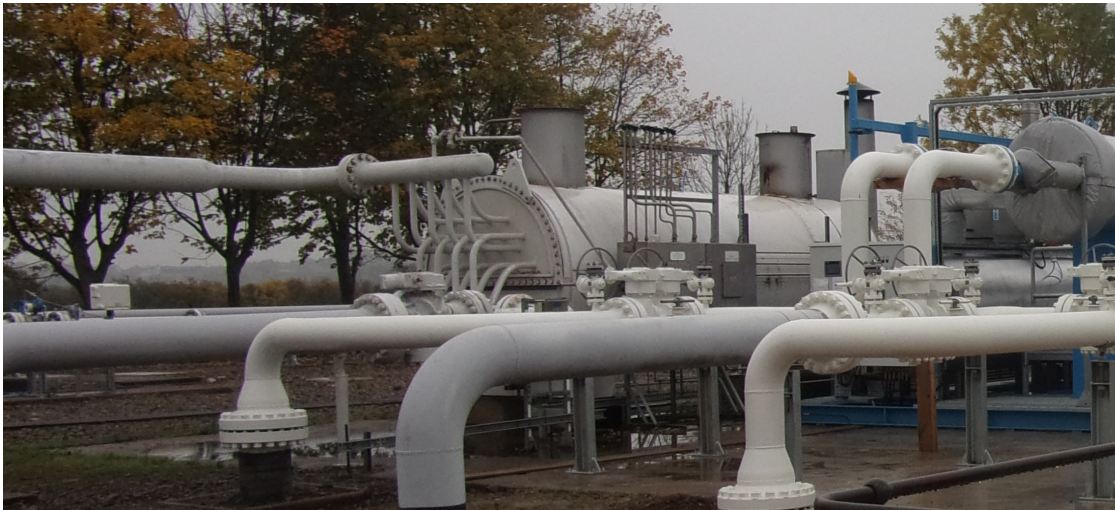
Figure 9. Retained preheating at Little Burdon providing an emergency back up only
