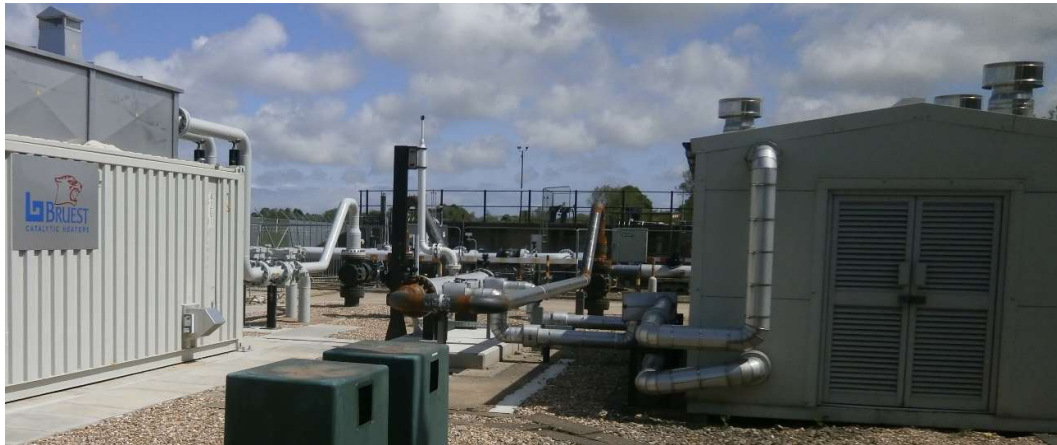
Figure 6. Retained preheating at Ganstead providing an emergency backup only
