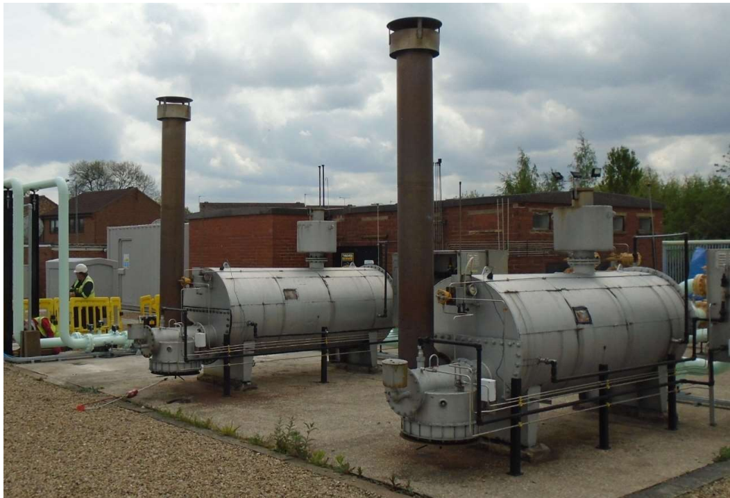
Figure 4. Retained preheating at Knottingley providing an emergency backup only
