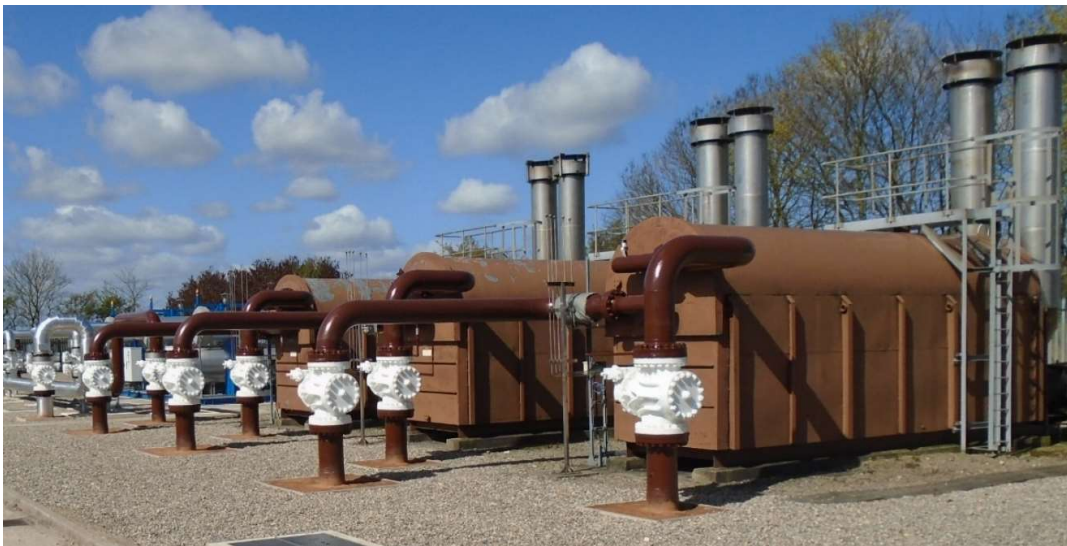
Figure 11. Retained preheating at Towton providing an emergency backup only
