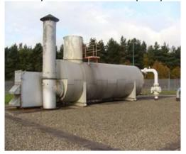
Operation of the units is simple as the burners are usually either 'on' or 'off'. Variances occur where some WBHs have 2 or 3 burners and some burners have 'high' and 'low' fire. WBHs are usually installed in pairs with one WBH capable of providing sufficient energy to
